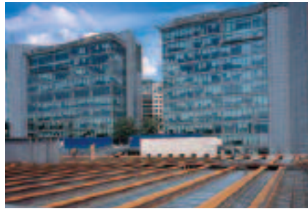
◀ The Crossrail Deck provides horizontal separation between PaddingtonCentral and the proposed Crossrail project
