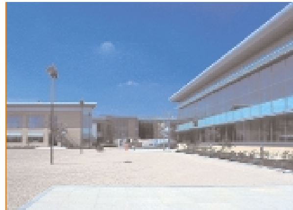
Cambourne Business Park
